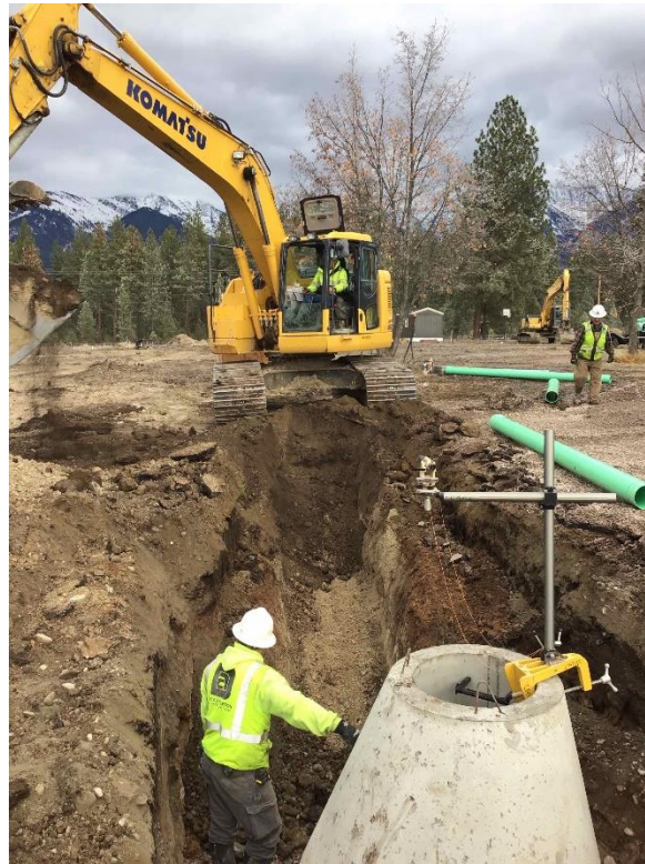
Kicking Horse Water and Wastewater Lines Replacement Project – 2020
